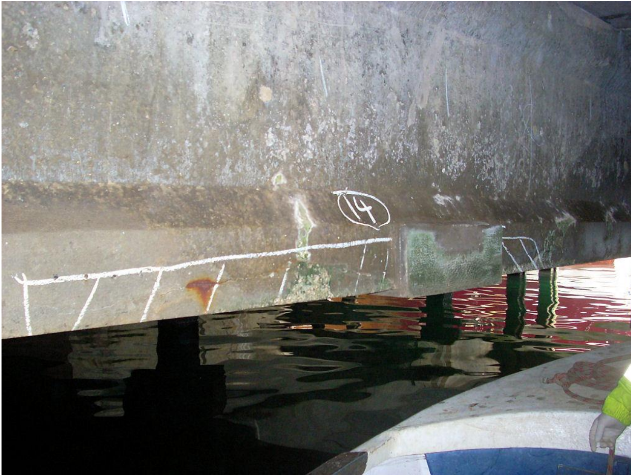
Example of 'Incipient Anode' Effect
