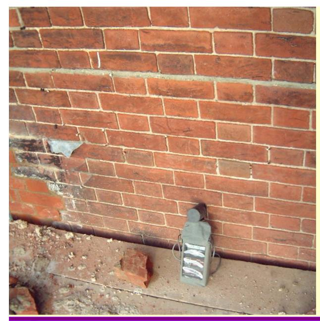
Cover Meter used to find depth of steel band which was jacking up brick courses
